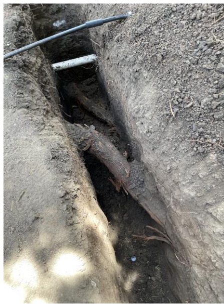
Significant roots in Southern and Western portion of the ADU exploratory trench
