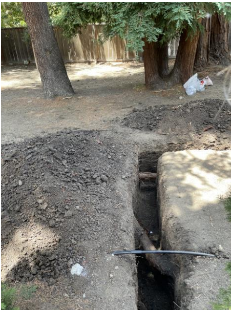
Significant roots in Southern and Western portion of the ADU exploratory trench
